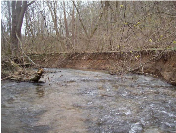
Figure 8. Elks Run streambank erosion (Site A) near the confluence with the Potomac River
